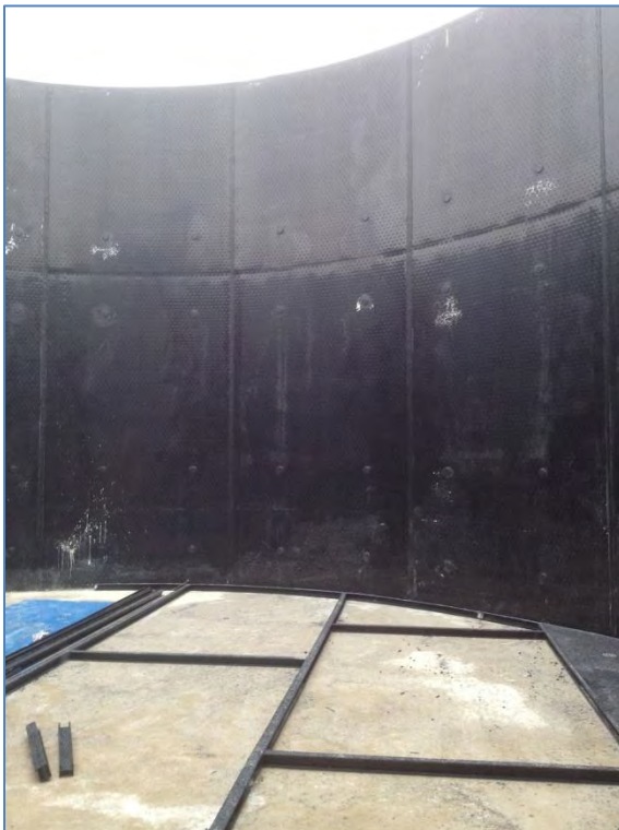
(Example: Floor lining using the AGRU I-Profile)
